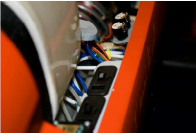
Photos 36 and 37 – left side – receiver batteries, switches and air gauges
